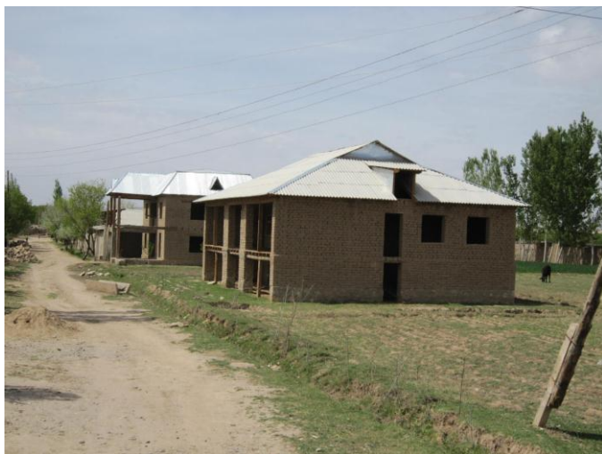
New houses being built by returning migrants from Russia. Jamoat Sayed, near Shaartuz (8 April 2011).
