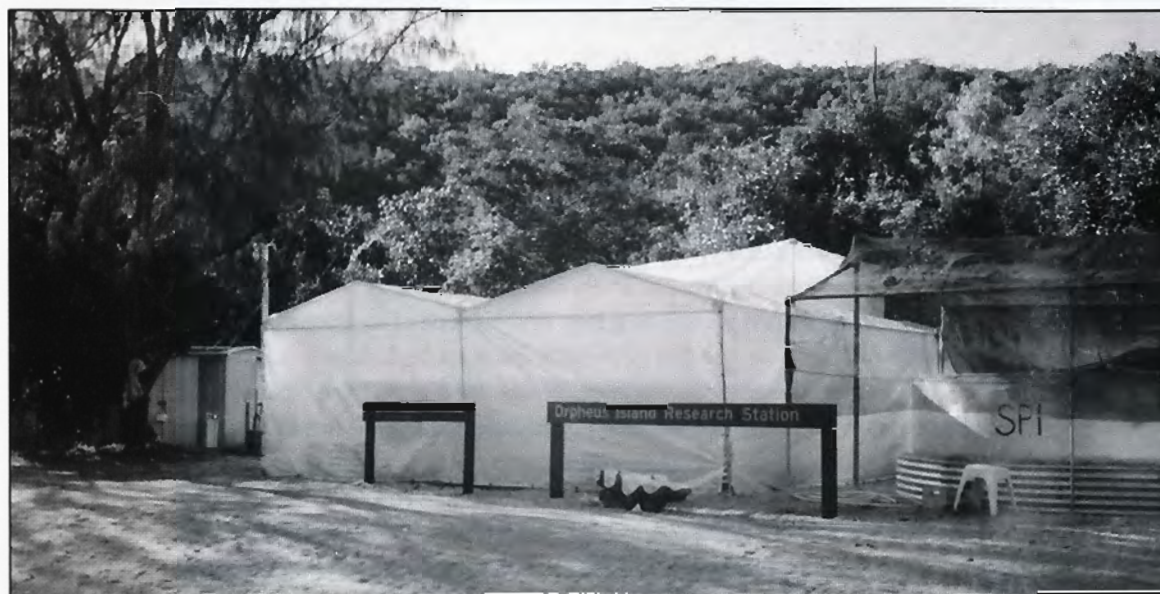
Figure 9.1 Greenhouse enclosure using 50% solar transmitting reinforced plastic material, JCUOIRS
