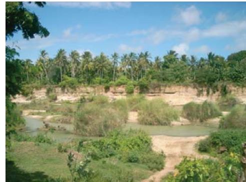
Bank erosion threatening coconut trees and surface water flow towards the river bed.
