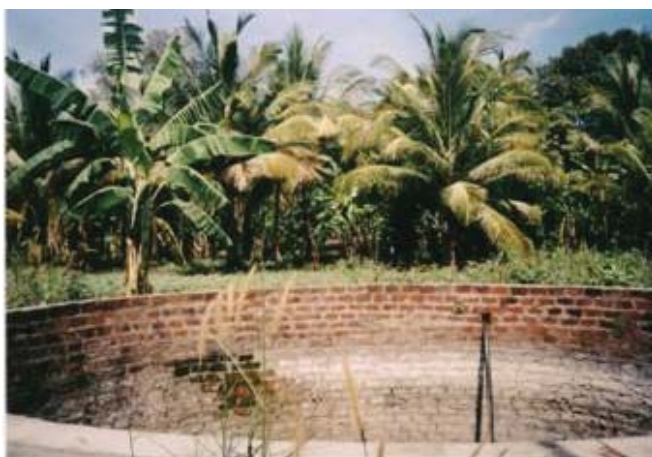
Figure 1. A large diameter agro-well with coconut trees in the background.
