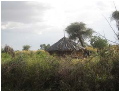
Figure 2: Geo-membrane used as roofing material, Alamata Socio-economic factors
