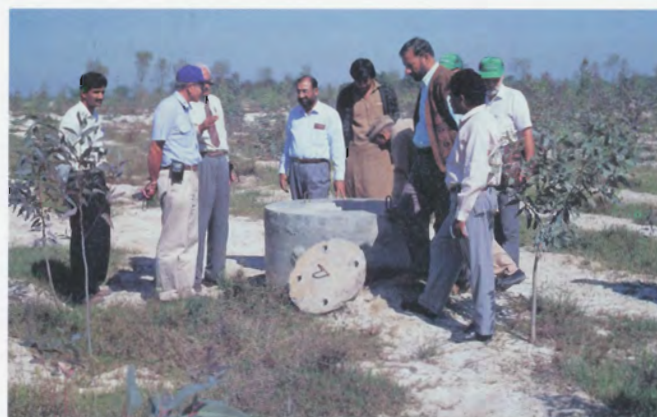
Photo 2.1. People gathered around a tile drainage access point. The land in this area has poor permeability to water and remained saline after tile drains were installed. [PHOTOGRAPH: E. BARRETT-LENNARD]
