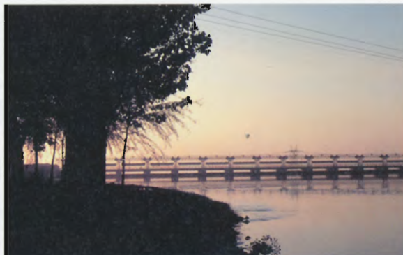
Photo 1.1. Balloki Head Works on the Ravi River. [PHOTOGRAPH: E. BARRETT-LENNARD]
