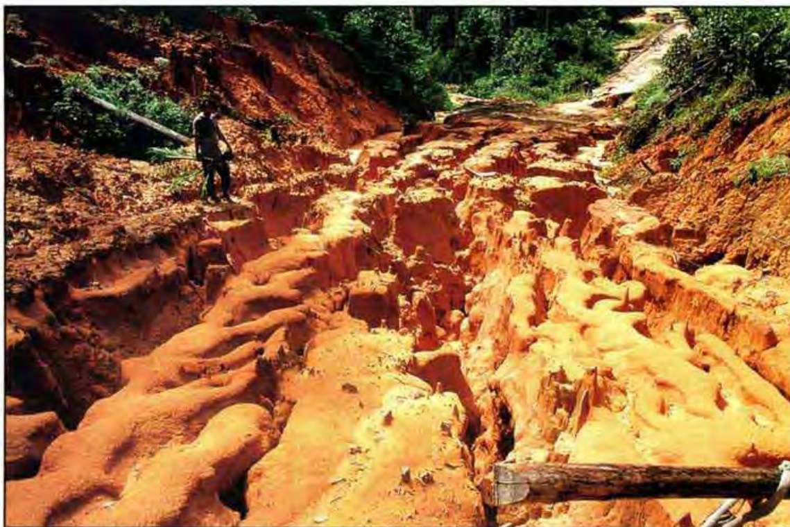
Heavy erosion is often observed on poorly-drained roads, especially where erodible sub-soil is exposed in steep road sections. (Photo: T.C. Whitmore)
