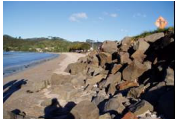
Figure 1 - Frontal seawall at Buffalo beach
