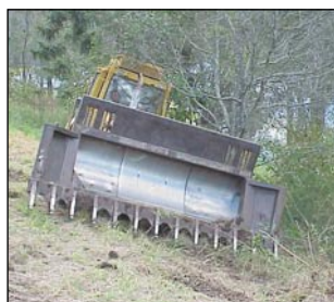
Figure 19. Mechanical clearing of lantana using a modified bulldozer (Queensland, Australia).
