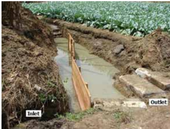
FIGURE 8. Pond with hardwood baffle.
