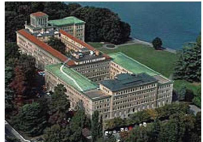
WTO building, Geneva, Switzerland
