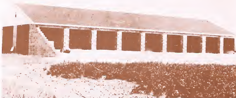
Figure 2.--In this modern storage (shown here before the earth bank was put in place) a 3-ton air conditioner supplemented the ventilation system (Storage No. 2).
