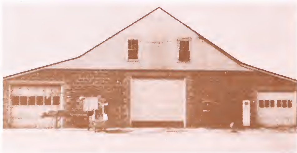
Figure 6.--In this storage, utilizing natural ventilation and free convection, cooling depends upon manual regulation of windows, doors, and ventilating ports. Storage temperature cannot be properly controlled (Storage No. 5).
