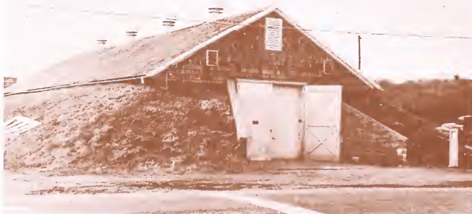
Figure 3.--This storage when filled has adequate refrigerating capacity to reduce potato temperature from 60 0 to 40 0 F. within 10 to 12 days (Storage No. 3).
