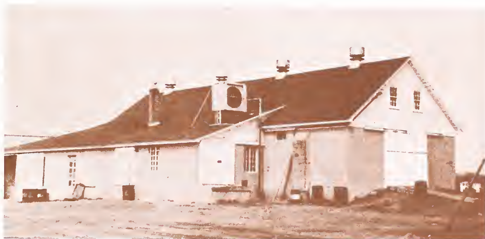
Figure 7.--The 15-ton refrigeration unit in this storage cools the potatoes rapidly but is used infrequently because of high operating costs (Storage No. 6).
