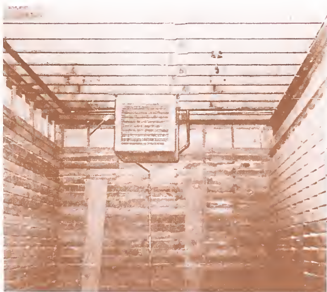
Figure 8.--The blast coil in this room cools the air overhead. Flow of heat from the potatoes to the air is accomplished by free convection (From Storage No. 6).
