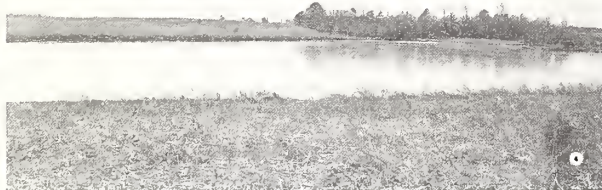
FIGURE 44.—Oxidation pond used for treatment of sewage and waste from a poultry-processing plant.
