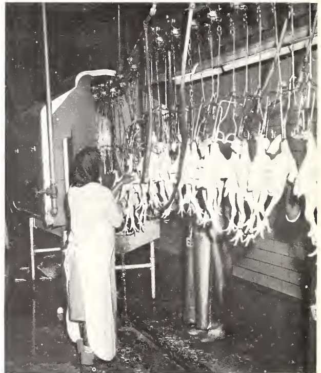
FIGURE 16.—Commercially processed broilers are conveyed through an "outside" bird washer (in the background) after they have been inspected for pinfeathers and singed.
