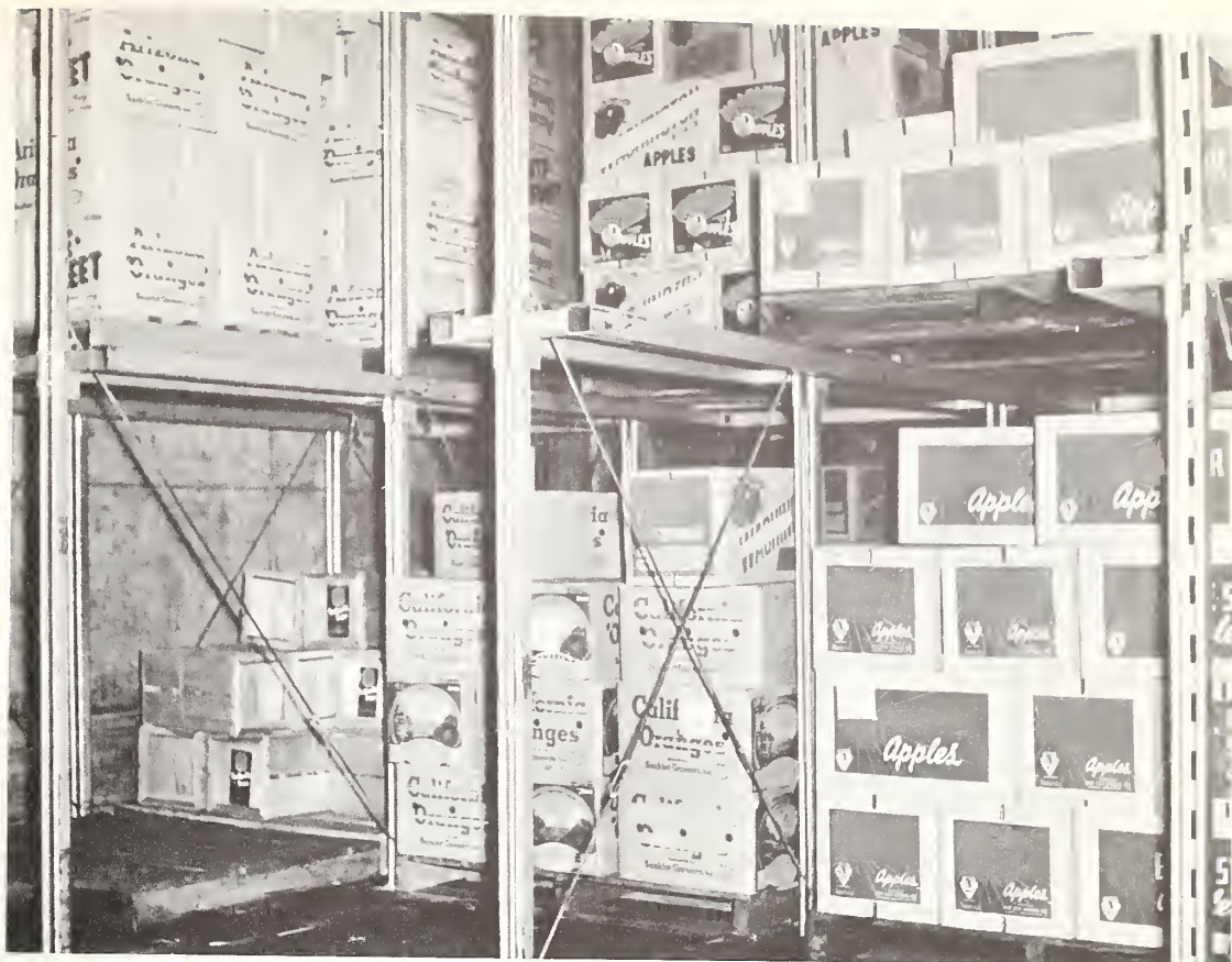
Figure 1.--The drive-in type of produce rack used with method A. The rack shown has a depth of three pallets. Each pallet-load of merchandise rests on individual supports.
