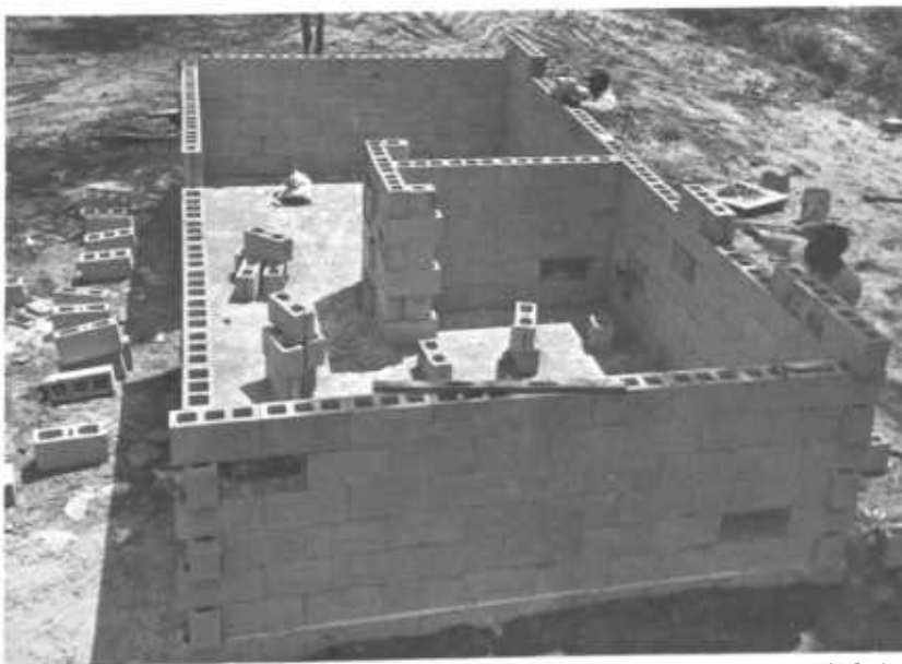
Dry stacking of concrete block walls for migrant labor quarters at John's Island, South Carolina.
