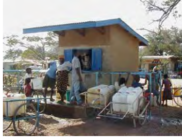
Figure 4. Tanzania. Top three photos: The Uchama water treatment plant and distribution kiosks responded to the town's growth as a result of mining. The program built community capacity and capability, and meant the company left a positive legacy.
