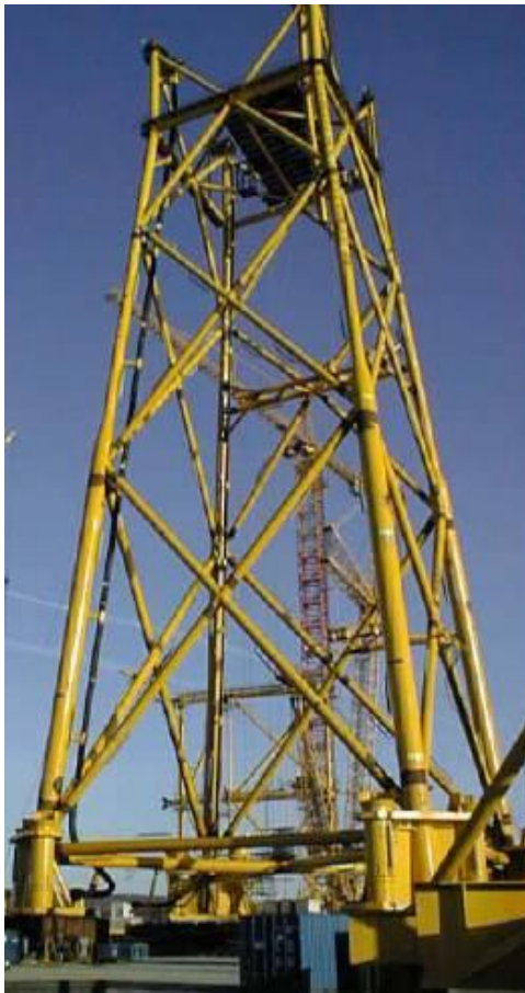
Figure 1. Steel jacket produced by Aker Verdal for a North Sea application (illustrative photo of a similar project completed previously)
