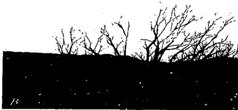
Roosevelt Reservoir, Salt River, Ariz.: A , Remnant of fill held between branches of tree and indicating former height of sediment deposits. B , Sediment deposits around large cottonwood trees; trunks entirely buried, branches only showing above surface.
