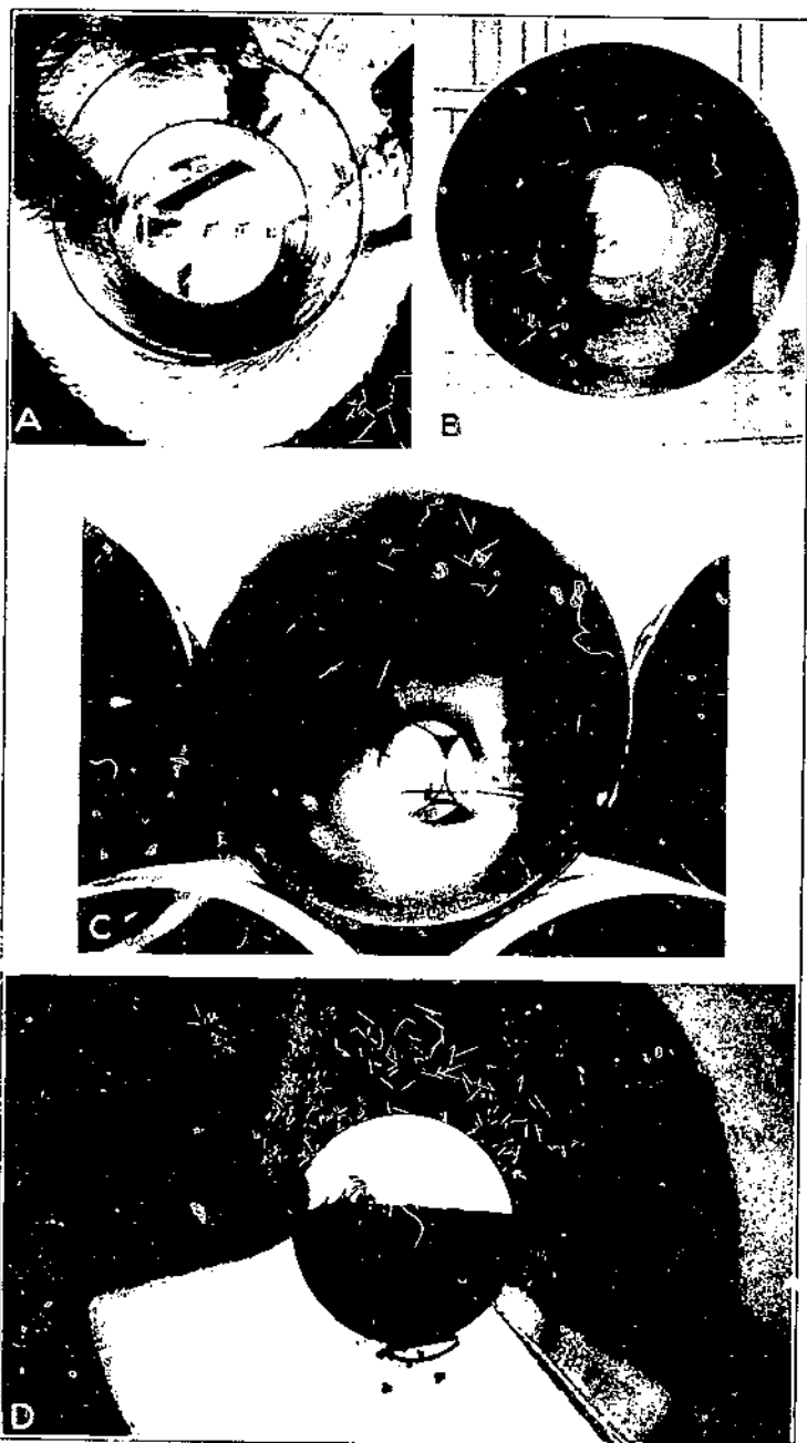
A - New direct and irrigation pipe. Top joint, looking up just direction of flow. B - New spiral belt joint pipe. End welded, top and field joints. Continuous interior. C - New lock for pipes in Princeton, Calif., 36 inches in diameter. Surface is smooth and glossy. D - New gatters for pipes in Bayview, California. Note welded troughs and rivets for girth screw, 6 inches in diameter. Note glossy mat when gatter is closed.
