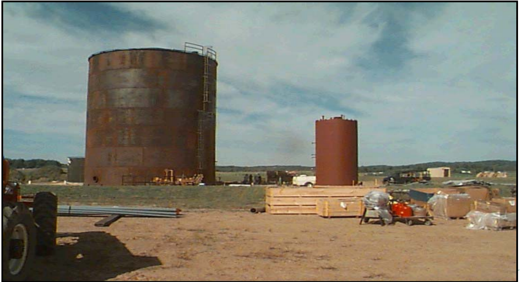
Digester tank and substrate tank
