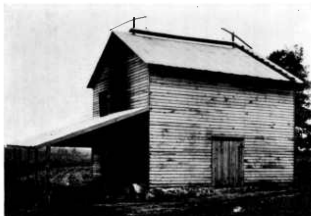
FIGURE 16.—Barn used for flue curing of tobacco is fitted with a good roof ventilator and ports in the foundation.
