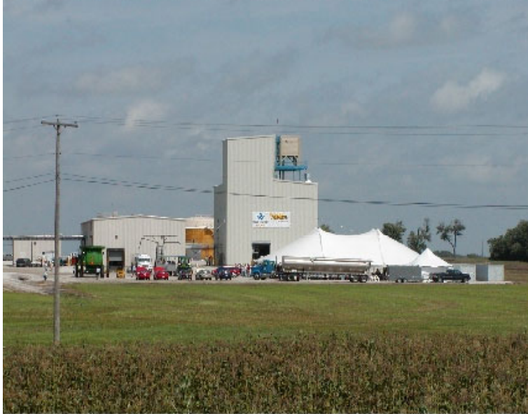
Figure 3. West Central Soy Biodiesel Plant
