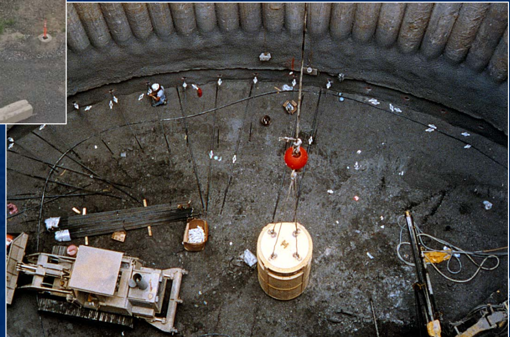
Secant Piles Shaft
