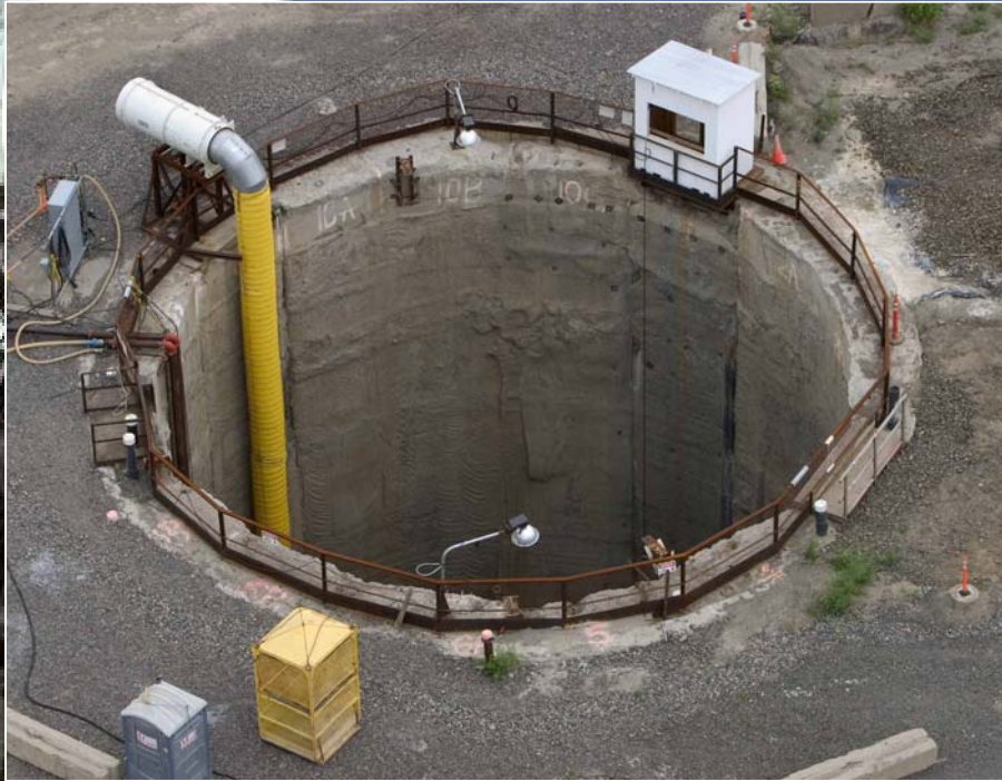
Slurry Wall Shaft
