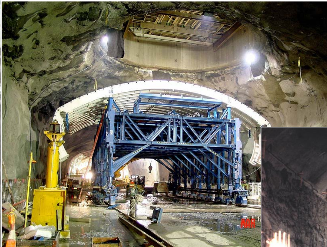
Weehawken Station HBLRT
