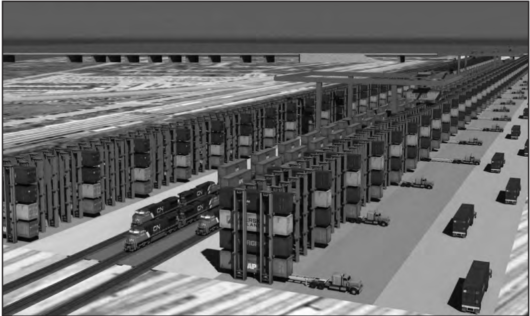
Figure 5: A Ramp With Vertical ATMS Stations
