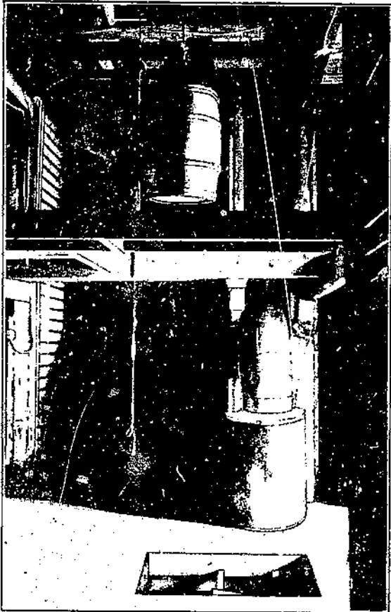
FIGURE 4.—Intermediate alley floor, experimental heater-ventilator (right), double-slatted bin partitions (at left), and barrel hoist.
