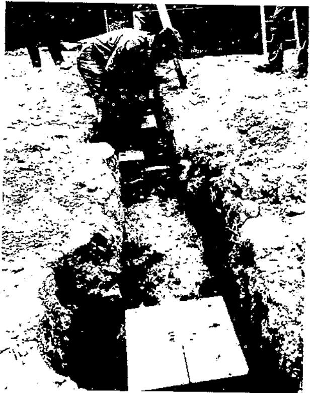
FIGURE 3.—Continuous ditch around perimeter of house.
