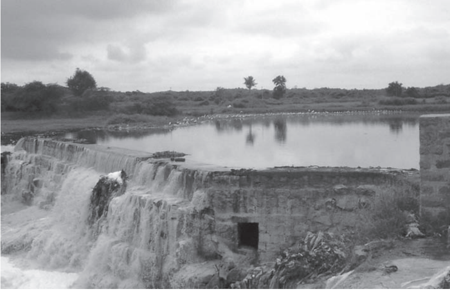
Figure 10.4 Weir in the Musi river, downstream of Hyderabad, Andhra Pradesh, India
