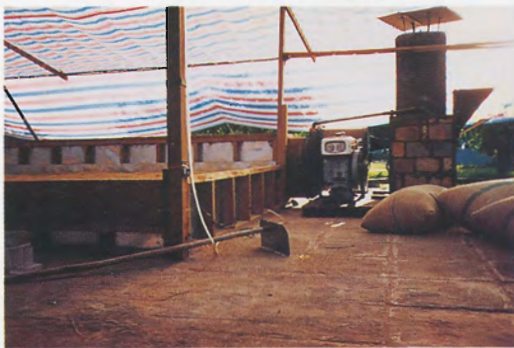
Figure 3. The new SHG-4 flat-bed dryer.
