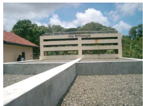
Community water supply scheme at Ariyagama, The tubewell at this place is 30 m deep from the surface level.
