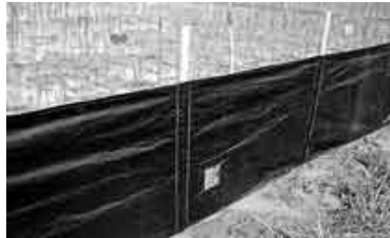
Figure 3.6 Plastic fence supported by bamboo posts.
