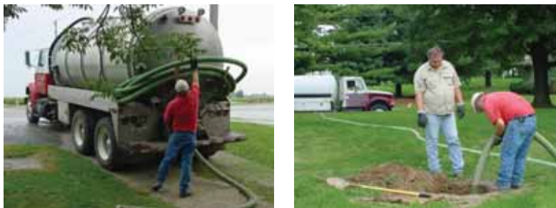
Figure 5. Emptying of the Septic Tank
